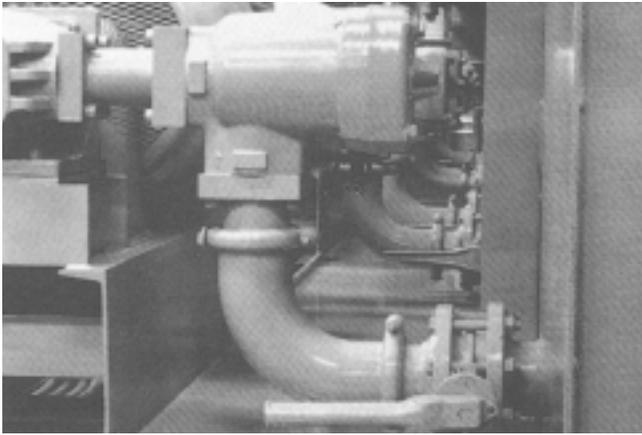
Flexmaster® joint elbows on a large hydraulic power system, which connect pipe from pumps to hydraulic fluid reservoirs.
